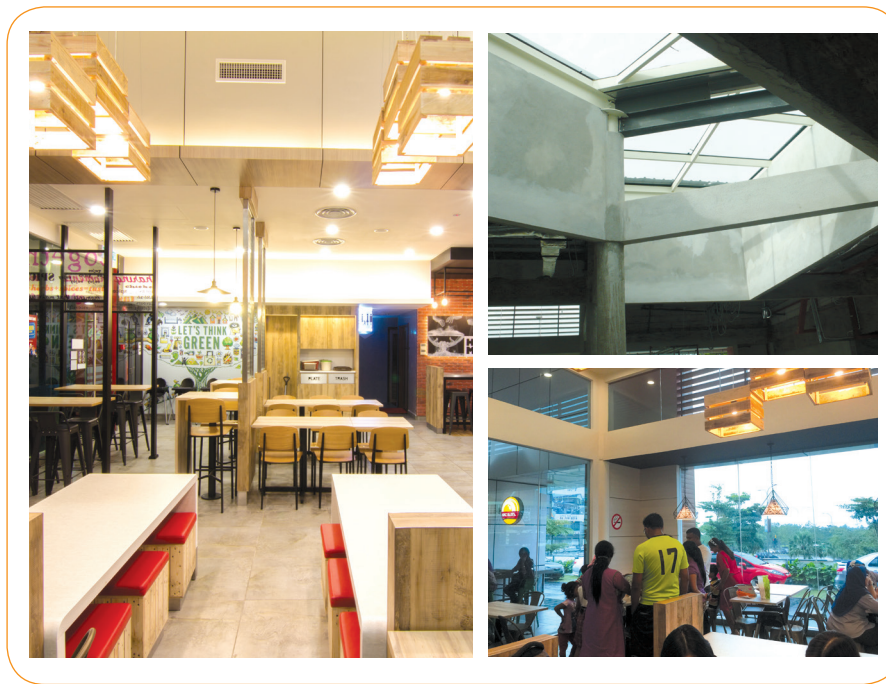
Lighting designed to meet the illumination parameters as stipulated under CP 38 (or equivalent) helps to achieve a good balance between comfort and energy efficiency. The restaurant is also designed with large floor-to-ceiling glazed windows and skylights, with low-e value, allowing natural daylight harvesting throughout the day. Images by Martin Lim.
