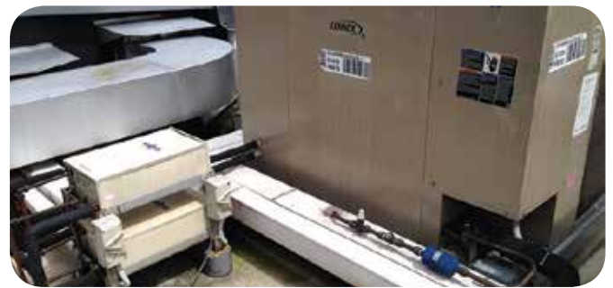
The Lennox HWL21/65 water heater module produces hot water from the waste heat generated by the air-conditioning units.
