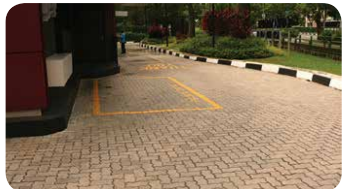
Recycled concrete has been used for pavement construction.
